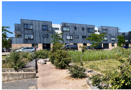
Our teams learn about rainwater harvesting systems at Clay Farm
