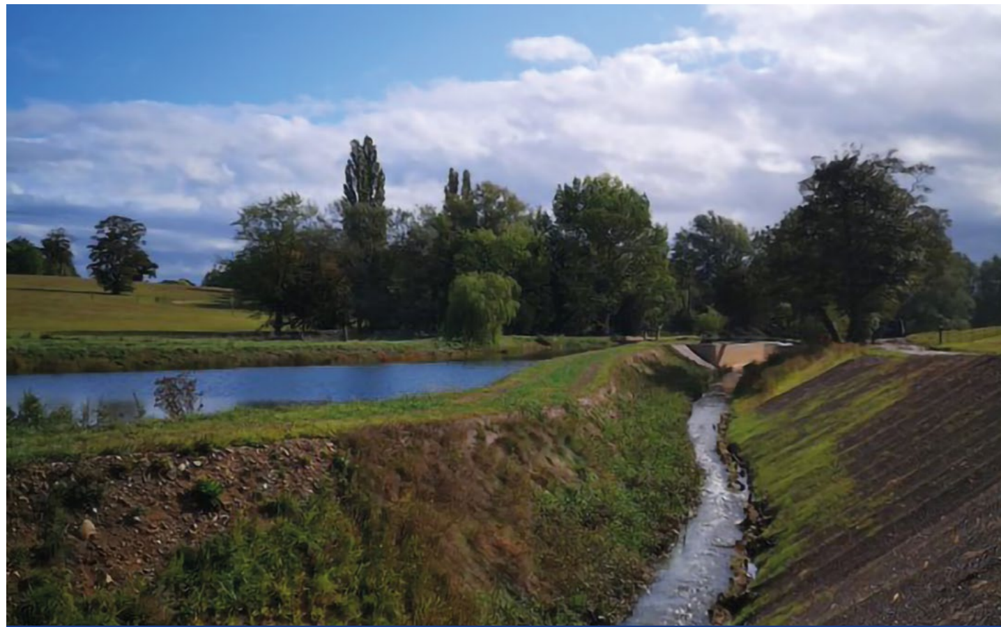
Construction of bypass channel on the River Beane
