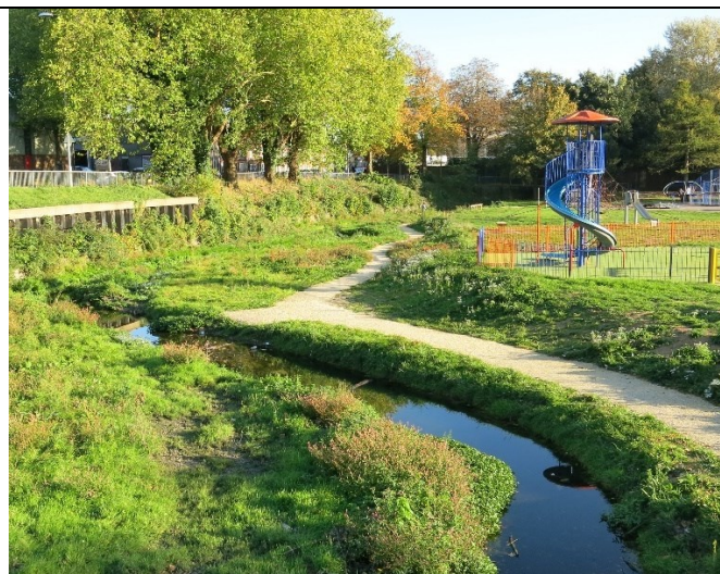
Figure 41: Post river restoration at Manor Road Park (September 2018)
