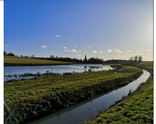
Figure 44: Live bypass channel adjacent to the Broadwater after completion of phase 2 of the Woodhall project (December 2019)
