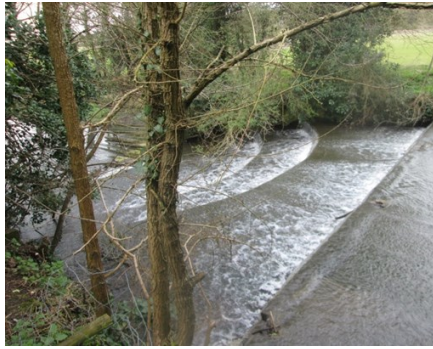
Figure 42: Horseshoe weir prior to phase 1 of the Woodhall project (2016)
