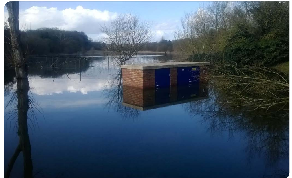
Figure 2-7 Flooding in 2014 prior to installation of site level flood defences
